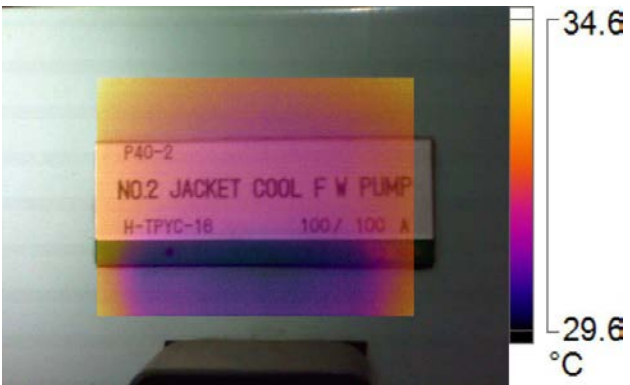
IR005118.IS2-No2 Jacket water pump 12/3/2016 8:50:46 AM
