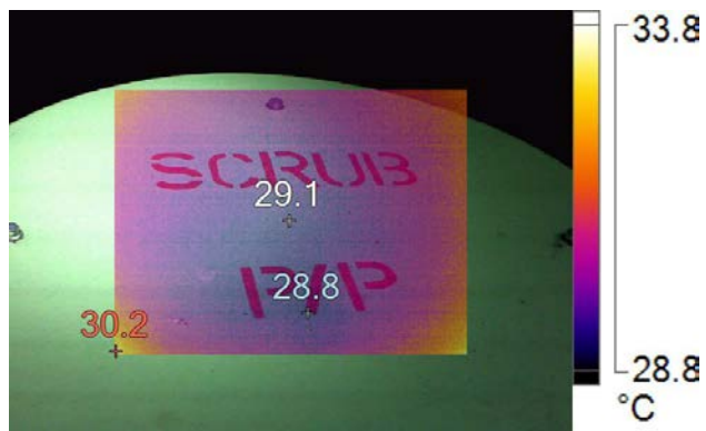
IR005172.IS2-Scrubber Pump 12/3/2016 11:18:18 AM
