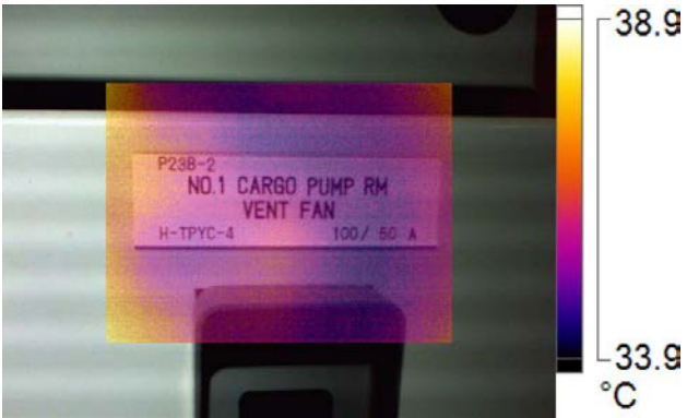
IR005964.IS2-No1 Pump room fan 12/6/2016 9:25:51 AM
