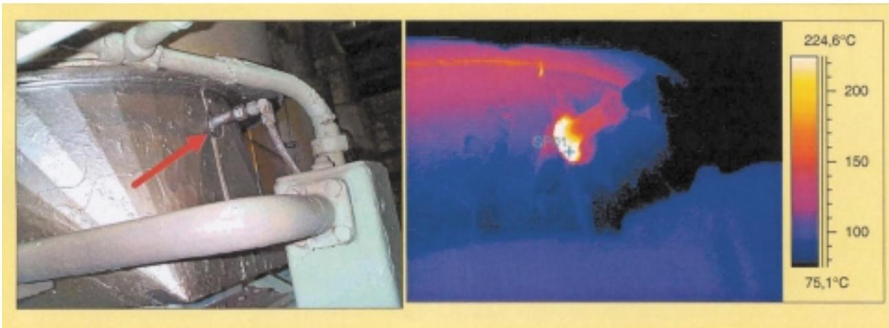
*Detail 4: Cut out for sensor. Insulation and steel cover to be applied tight to sensor pipe or in some cases along sensor pipe. Hot spot = 230°C.*
