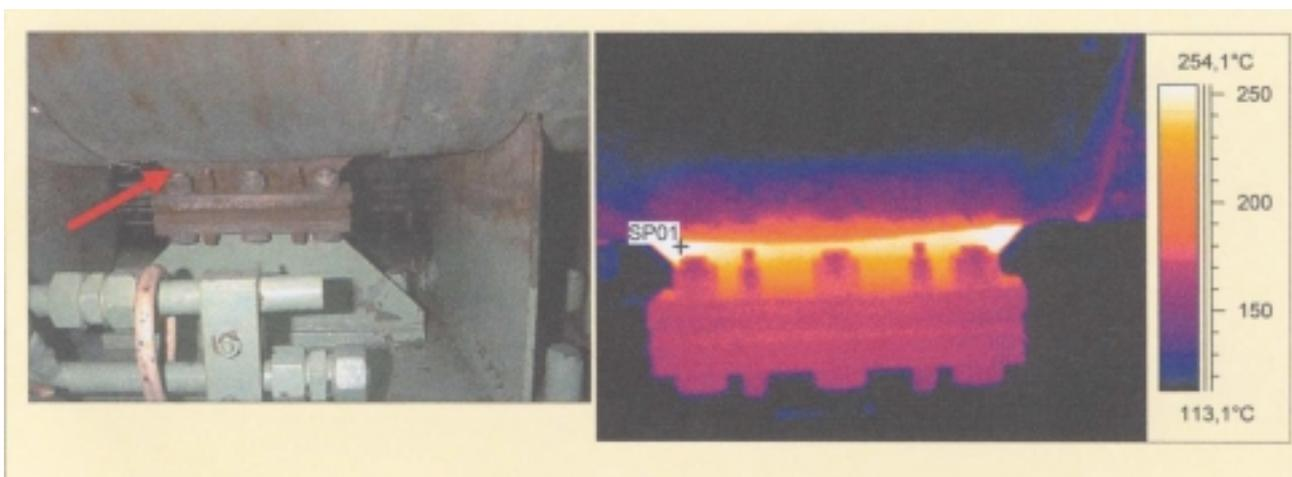
*Detail 5 – Foundation penetrates exhaust duct insulation. Flanges to be provided with insulation. Hot spot = 260°C.*
