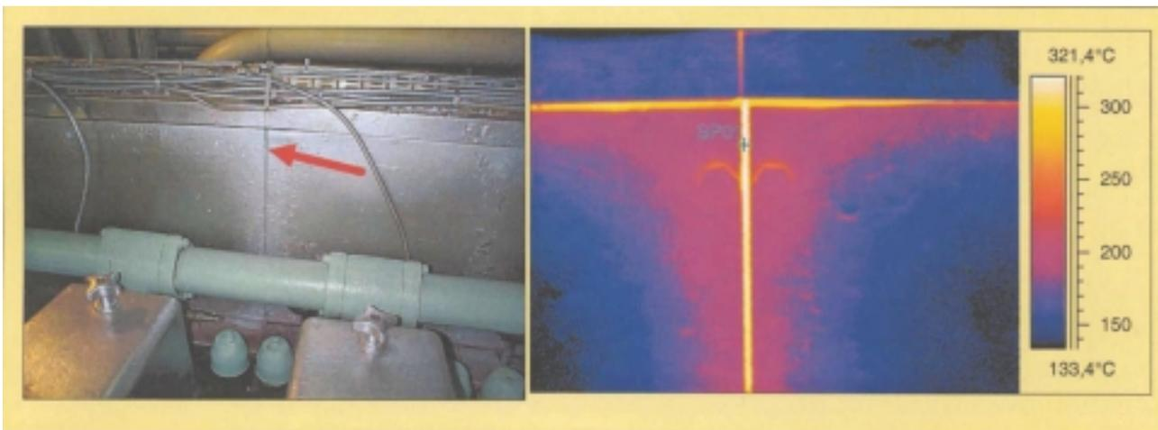
*Detail 2: No overlap between steel sheeting covering exhaust manifold. Same problem often found on "insulation pad" type insulation. Larger gaps in insulation than shown on above picture can often be found. New steel sheeting with proper overlap to be provided or additional protection to be applied in way of joints. Hot spot = 320°C.*
