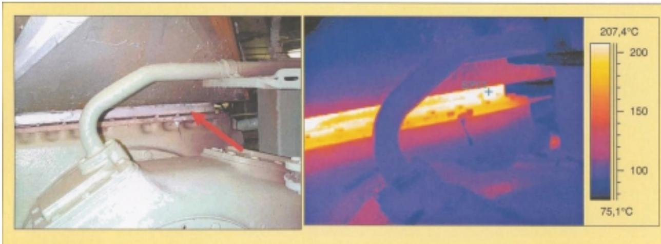
*Detail 3: No insulation of flanges between exhaust manifold and exhaust duct. Hot spot = 230°C.*
